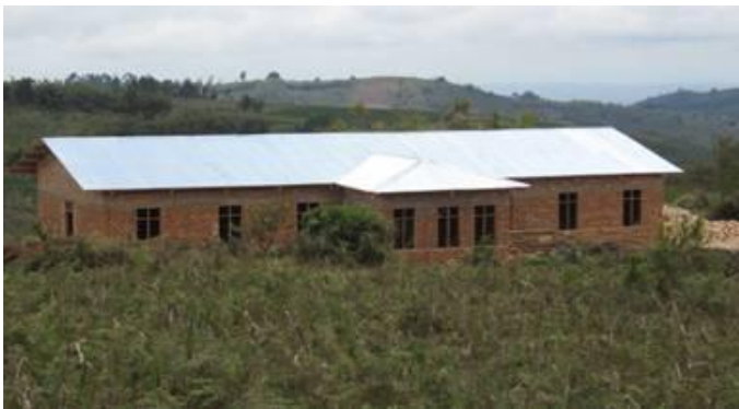
Back View of our new Dorm for Girls at Madisi. The wing in the middle is for the two dorm moms. The windows you see are for six more rooms.
